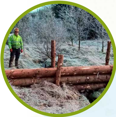
Installing woody debris flow restrictors, mimicking fallen trees, to hold back high flows
